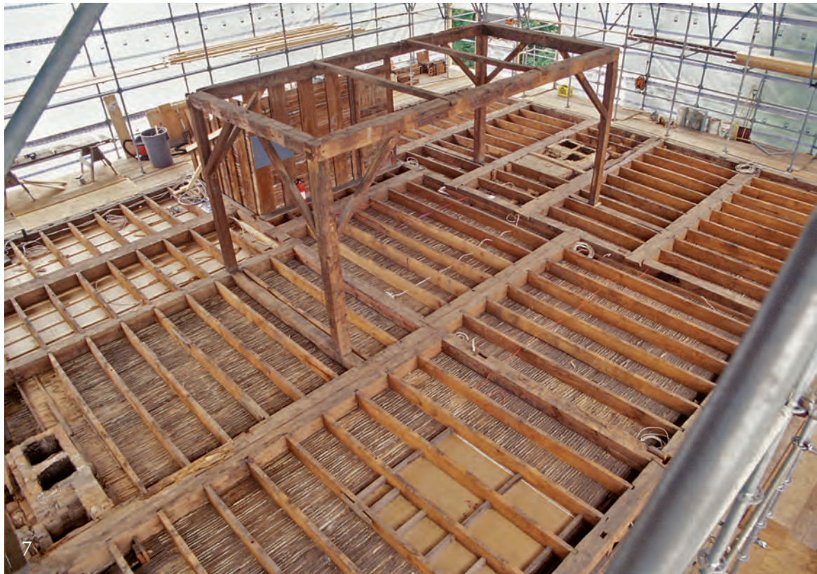
5 Full-length posted purlin system under 19th-century gable roof frame, 18th-century posted purlin assembly just visible inside. Wall plate on studs carried 19th-century rafters.
