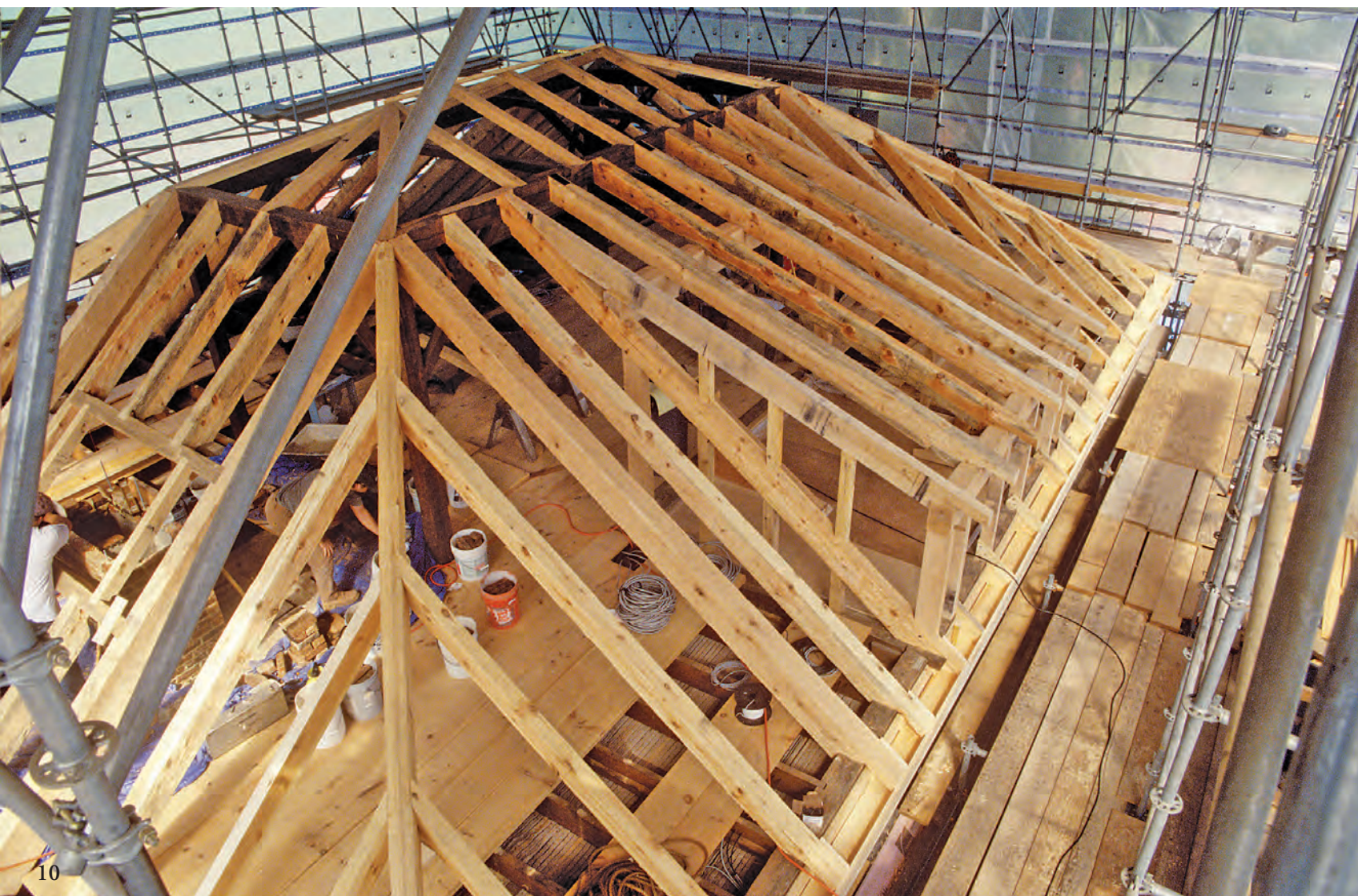
8 General Ashley House, Sheffield, Mass., two common rafters in place, hip rafter being scribe-fitted by Thomas Lanoue, 2002.
