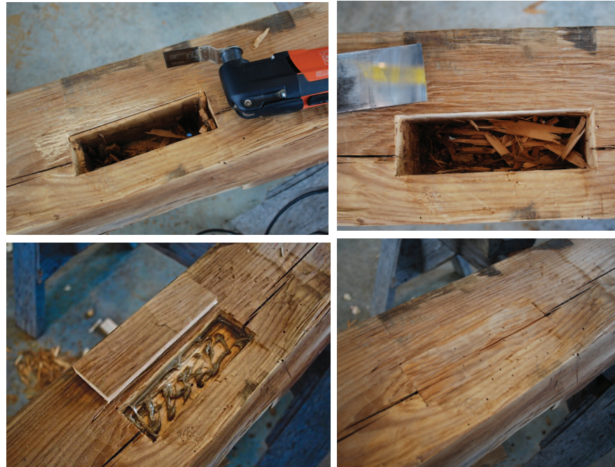
7 Partial sequence of patch prep after grain-match : a) trimming after knifing and roughing, b) deepening walls with framing chisel, c) setting filler block and glue, d) fitting patch.
